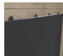
3. Fix screen on wall ;
